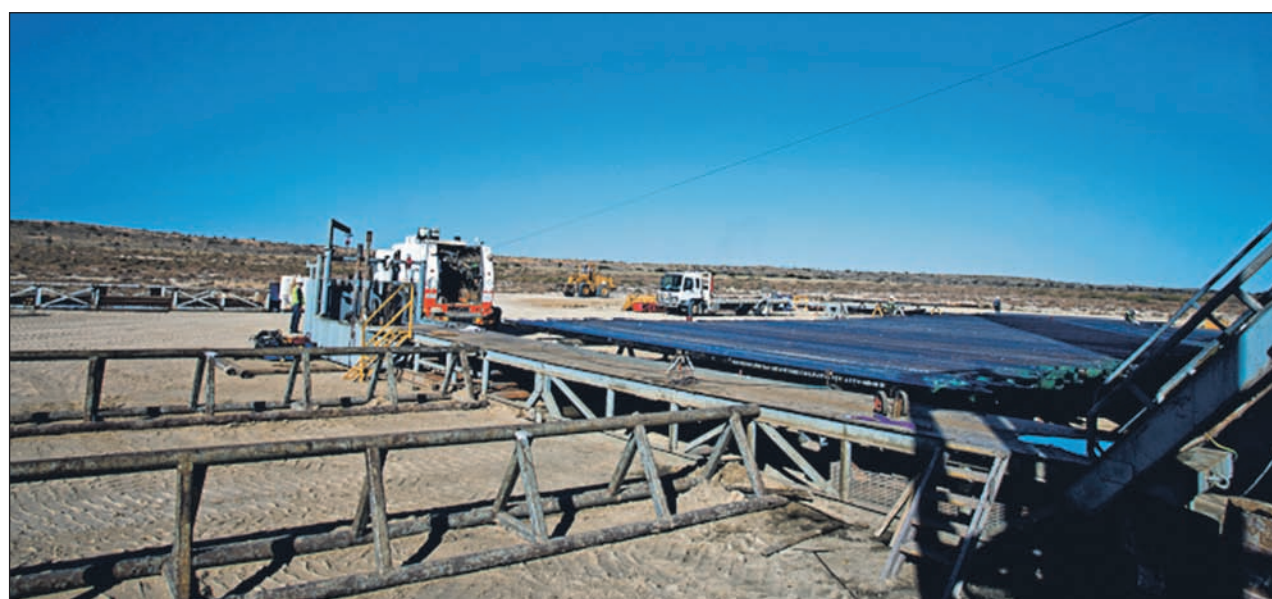
Casing at Snellings-1 drill site
